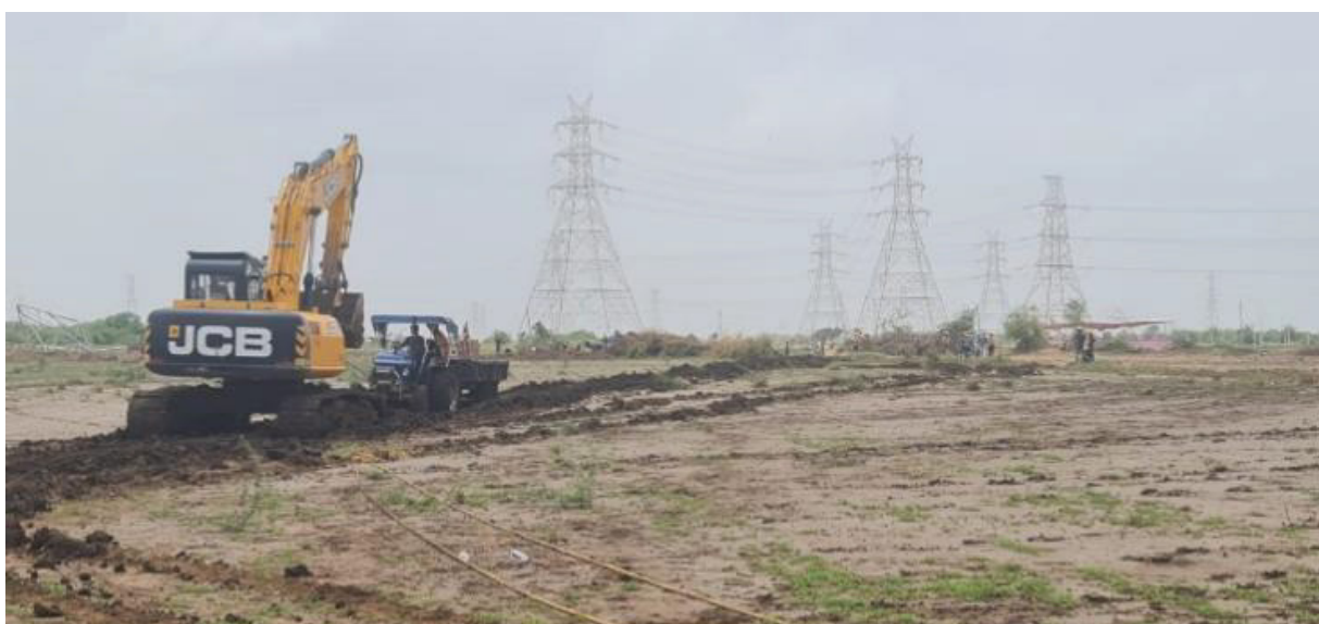
Figure 7.7: Use of Poclain Machine in Wet fields for material shifting
