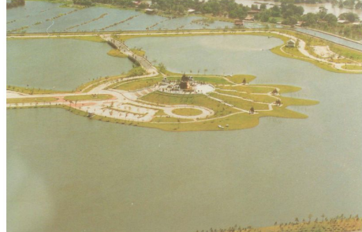
A royal park with flood-retention storage initiated by H.M. the King of Thailand in Ayutthaya Province in the lower Chao Phraya River Basin
