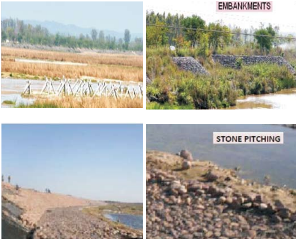
Figure 3: Photo graphs depicting structural mitigation measures viz. stone spurs, embankments, aprons and stone pitching.
