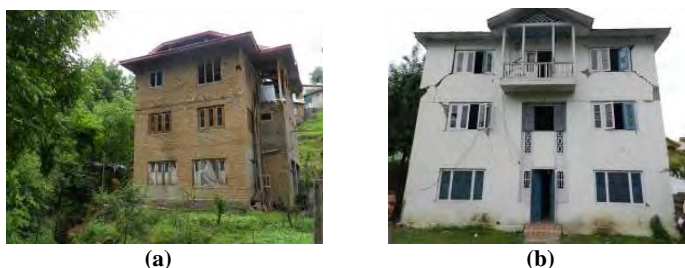
Figure 5: Brick masonry houses: (a) houses with RC floors did better even though they had no earthquake-resistant features like horizontal bands, and (b) houses with heavy wood floors did poorly; the walls dilated outwards in both plan directions and reduced the bearing of wood floors on the walls
