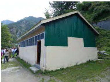
Figure 9: Wood frame single-storey school construction with brick masonry up to sill level and light roof
