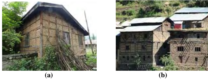
Figure 4: Variant of Dhajji-Dewari Houses: (a) without diagonal wood members, and (b) with no Dhajji (wood frame) in the ground storey
