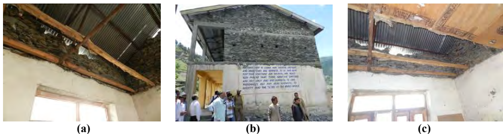
Figure 8: (a) Informal trusses rested directly on stone walls without any wall plates (at Gandoh), and (b) large stone gables not provided with gable bands and gable end trusses are not complete with bottom chord and vertical posts (at Bhalessa), and (c) falling of false ceiling due to poor anchorage
