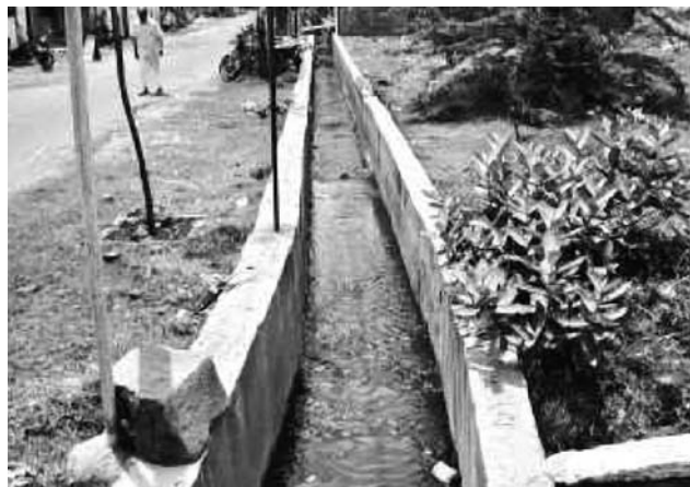
Storm water drain carrying sewage
