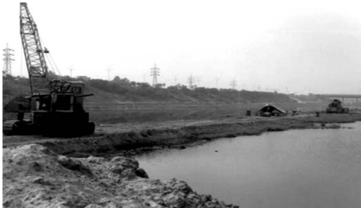
Figure 9 Desilting work going on at Najafgarh Drain.
