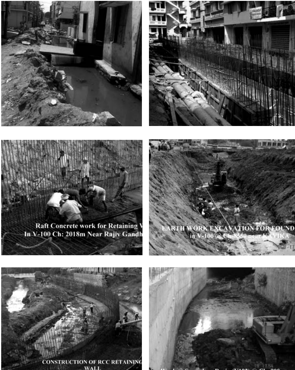
Plate 5.6: Construction of RCC box drain in Puttenahalli (Source: BMP)
