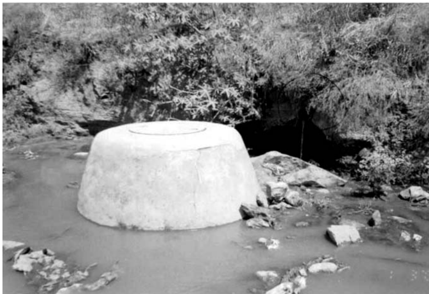
Plate 2.4: Manhole and a sewer connection – obstruction as well as pollution (Source: BWSSB)
