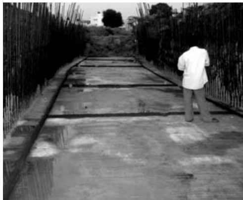
Plate 5.8: Storm water drain retaining wall construction (Source: BMP)
