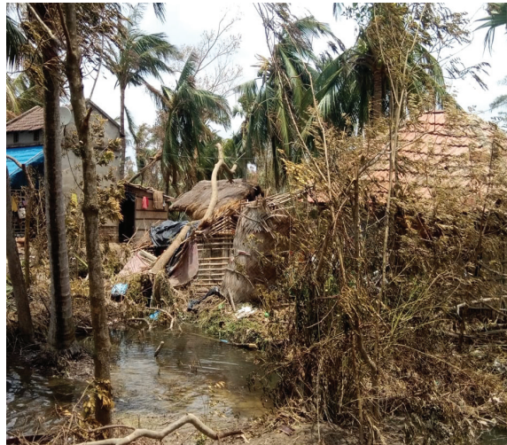
Figure 4: Houses Destroyed in Patharpratima, South 24 Parganas.
