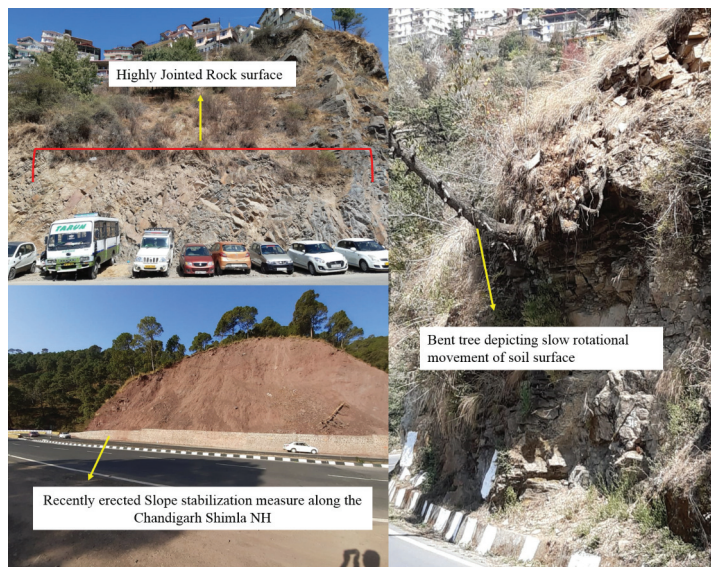
Figure 16: Settlements located along highly jointed rock surface; Soil slipping along the NH
