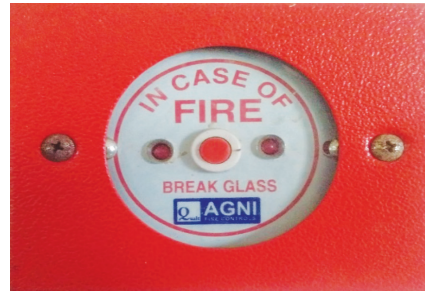
Figure 2 : (ii) Manual Fire Alarm System
