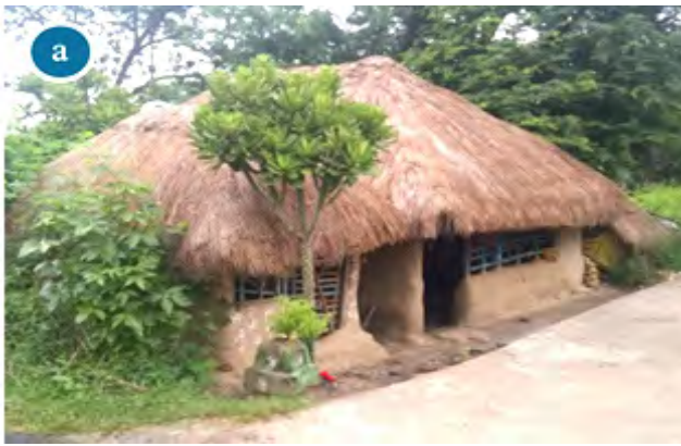
Figure 3.2: a) Mud house with thatched roof; b) Mud walls with tile roof supported by stilts
